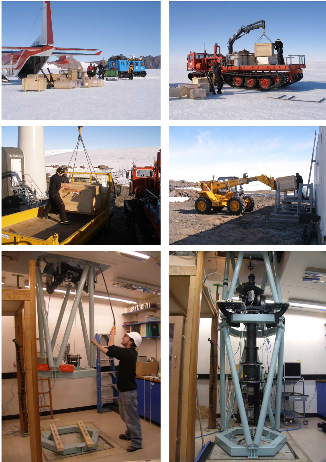
Figure 4.1.1: Sequence of images (ordered from top left to bottom right) showing the stages of installation of the Mawson SDI. They show, in order: boxes containing instrument parts unloaded from aircraft onto the Antarctic plateau; transfer of boxes onto a truck for transport to Mawson station; arrival of boxes at Mawson station and transfer onto a utility vehicle for transport to the Aeronomy building; unloading of boxes into the Aeronomy building; raising of the top-level frame to enable placement of lower-level frame beneath; the fully assembled instrument with optical components (suspended in the centre of the light-blue frame) shown in the lowered position. Images courtesy of Mr. Theo' Davies.
